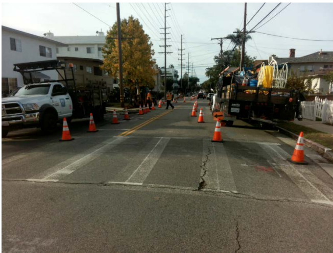
SCG Relocations Modified Traffic Control Along Ohio Avenue
