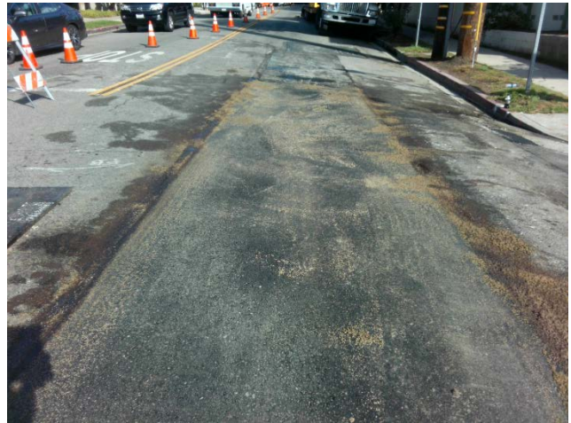
SCG Relocations Repaved Roadway Ohio Avenue and Butler Avenue
