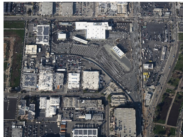
Division 16 - aerial photo
