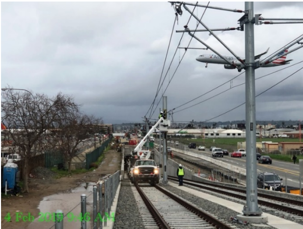
South end – Working on overhead line
