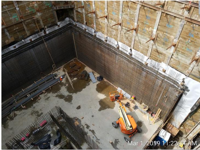
Rebar installation at Wall F in Historic Broadway Station
