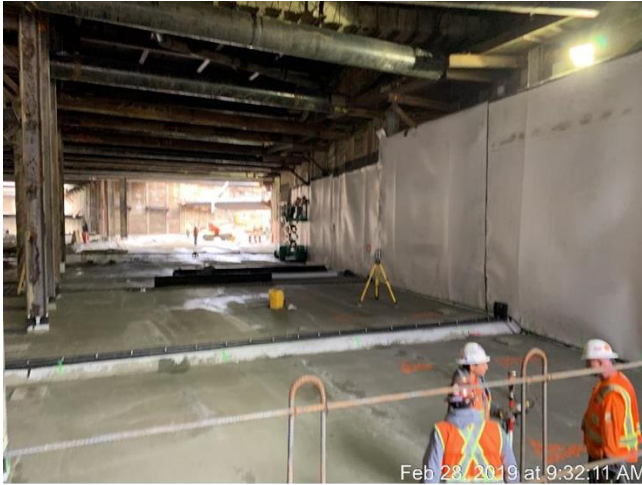
Protection slab placement at 1st/Alameda Wye
