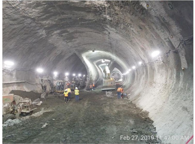
Right center wall demolition at SEM Cavern
