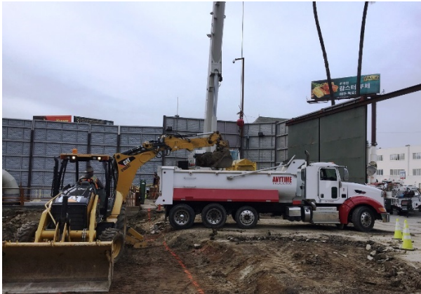
Excavation for Gantry Crane at Wilshire/Western
