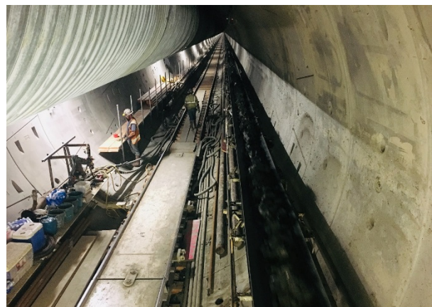
Reach 1 Tunnel Looking West
