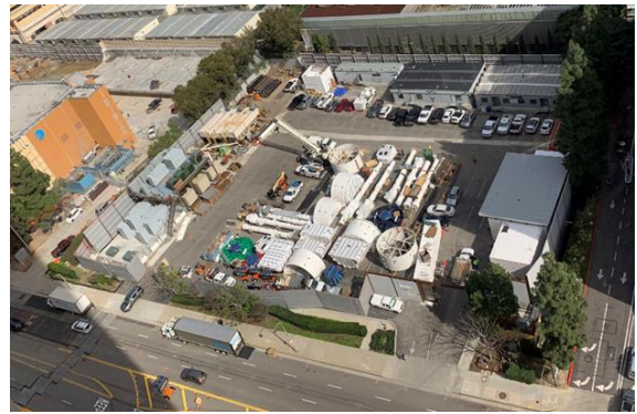
TBM Staging area in Century City
