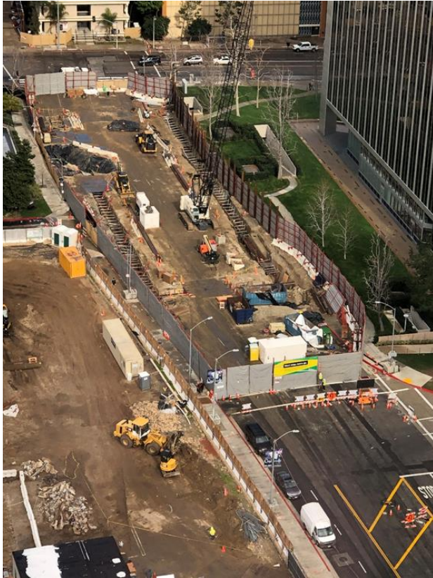
TBM Launch Box Overview in Century City
