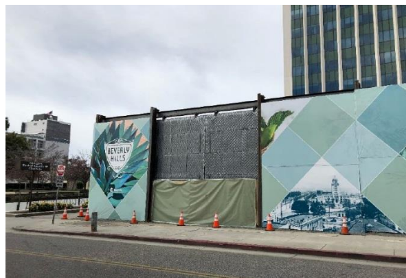
Gate Installation at Reeves in Beverly Hills
