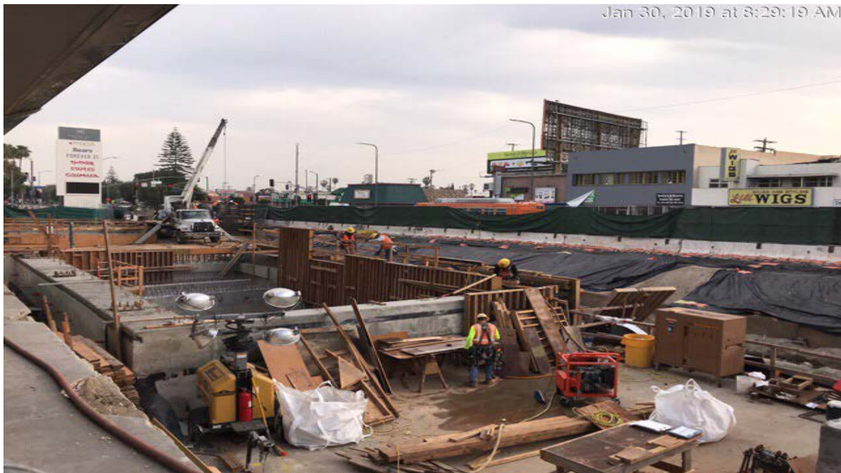
Plaza level walls at Martin Luther King Jr. Station
