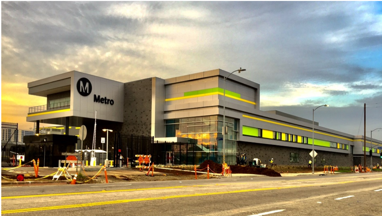
Main Shop at Southwestern Yard (Division 16)
