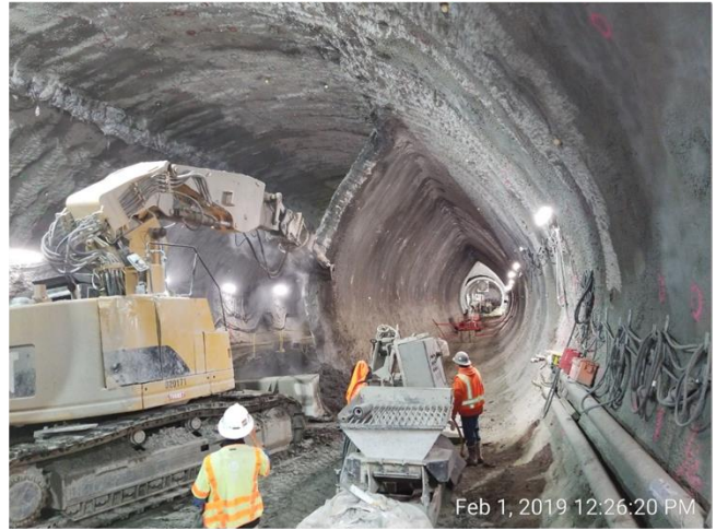
Right center wall demolition of SEM Cavern
