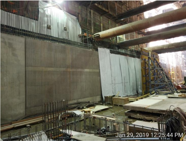
Wall D concrete curing in Historic Broadway Station
