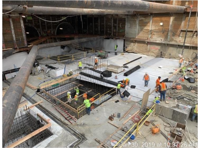
Sump/Ejector pit invert placement in future Little Tokyo/Arts District Station
