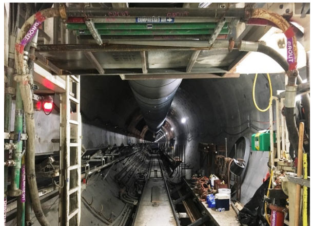
Reach 1 Tunnel Looking West
