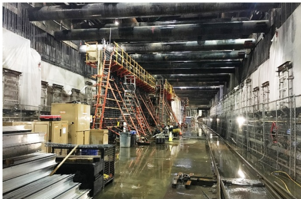
Wilshire/La Brea Station Looking East
