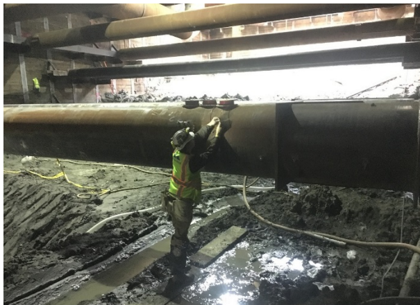
Strain Gauge Installation at Wilshire/La Cienega Station
