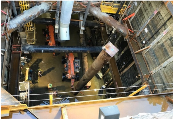
Lifting Strut out of the Wilshire/Western Shaft
