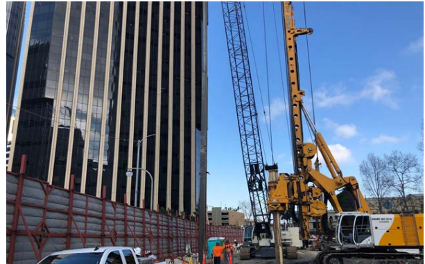
Soldier Pile Installation in Century City
