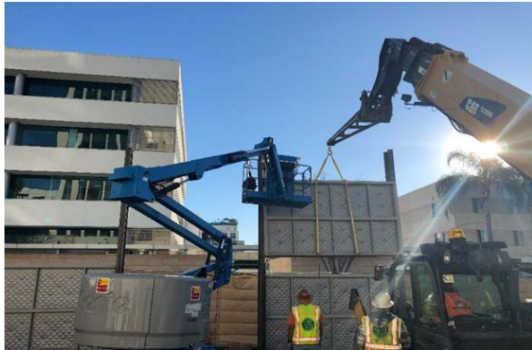
Sound Wall Installation at Reeves Staging Yard in Beverly Hills
