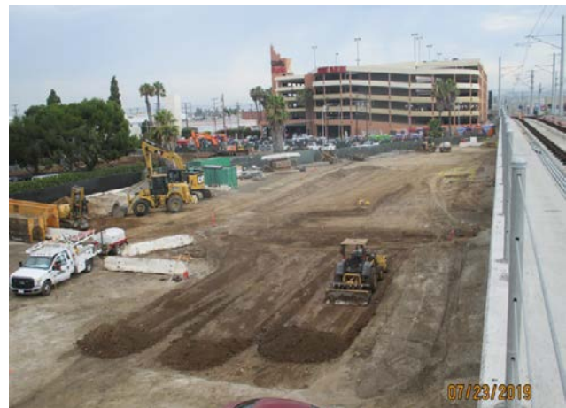
AVIATION/CENTURY STATION - Grading for the plaza and parking lot.
