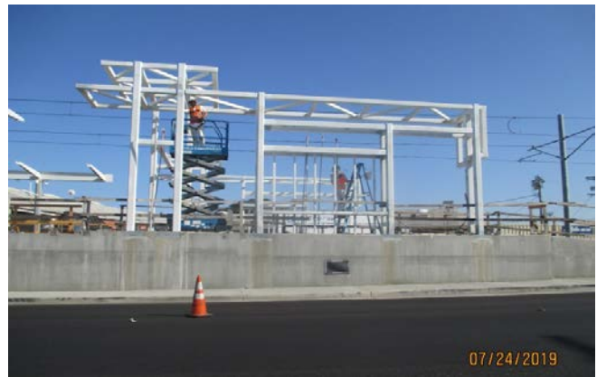
WESTCHESTER/VETERANS STATION – Placing the ticket vending machine structure.
