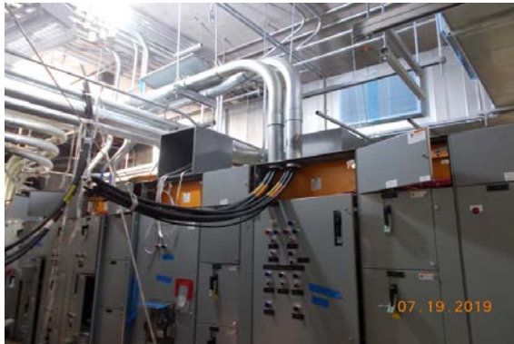
EXPOSITION/CRENSHAW STATION – Installing emergency fan cable feeds for Auxiliary Power Room.
