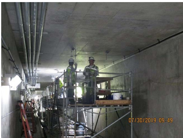
UG STRUCTURE #3 - Continued installation of overhead catenary rail brackets.
