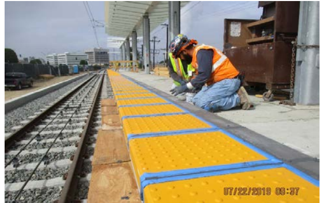
LA BREA STATION – Placing grout in yellow paver joints.
