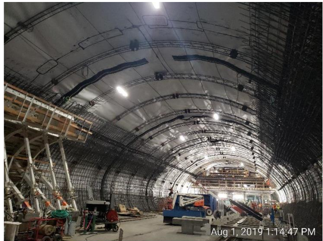
Back face rebar installation in SEM Cavern
