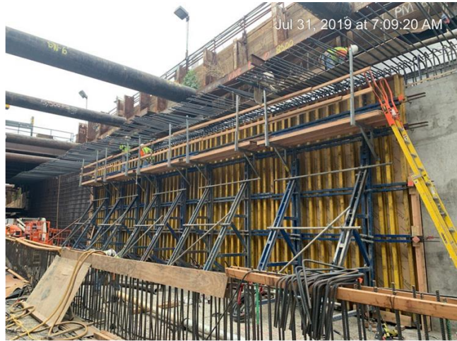
1st Street Cut and Cover exterior wall pour
