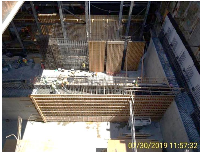
Concrete placement of interior wall at Historic Broadway Station
