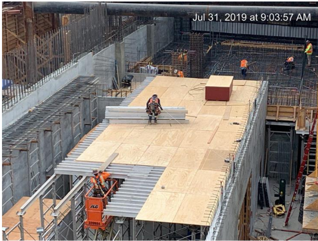
Future Little Tokyo/Arts District Station ancillary level deck installation
