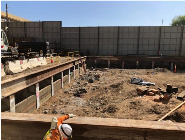
Tunnel Shaft Excavation in Century City
