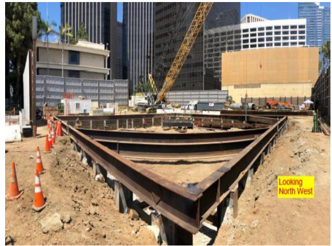
Tunnel Shaft Excavation in Century City
