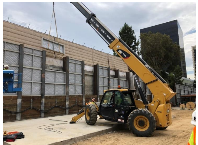
AT&T Staging Yard Sound Wall Pile Installation in Century City
