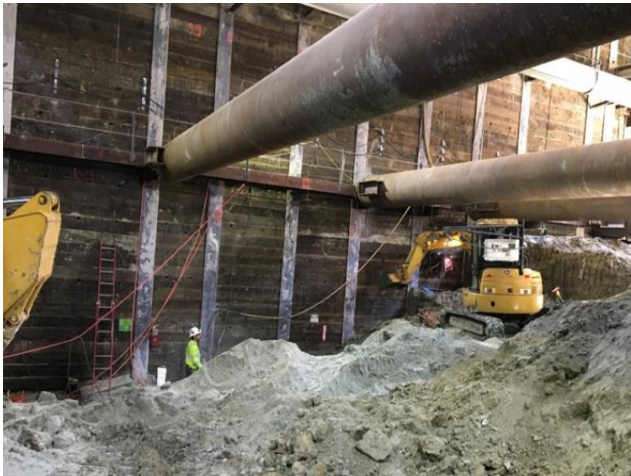
TBM Launch Box Excavation in Century City
