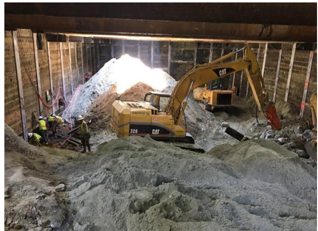
TBM Launch Box Excavation in Century City
