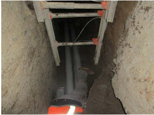
Installed 120' of 7-4" Conduits.
