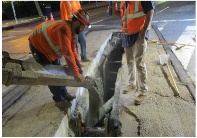
Backfill Slurry for Joint Trench for Fiber Optic Main Line
