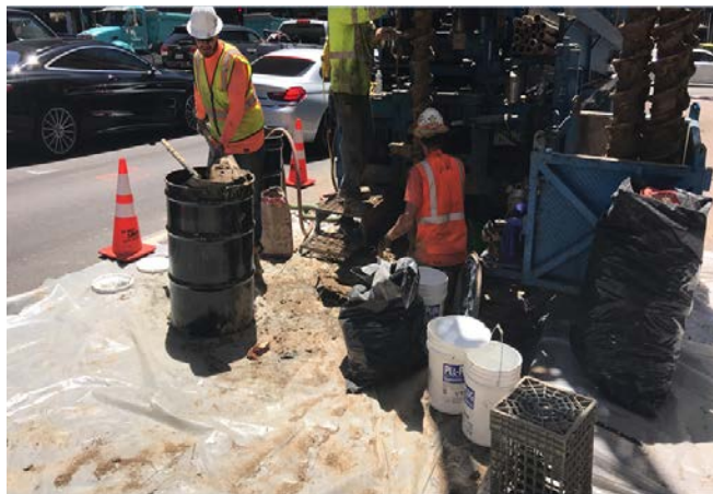
Geotechnical Boring for Tunnel Cross Passage Design on Wilshire Blvd.
