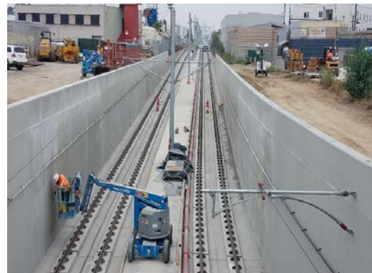
UG3 – Continued finish work on U-channel walls of southbound portal.
