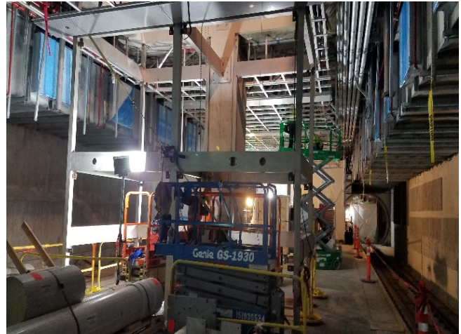
EXPOSITION/CRENSHAW STATION – Continued installation of elevator frames 3 & 4 at the platform level.
