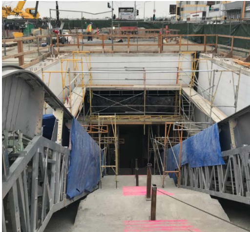
LEIMERT PARK STATION – Continued tile installation from mid-landing to plaza.
