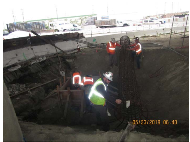
Setting rebar cage for C2
