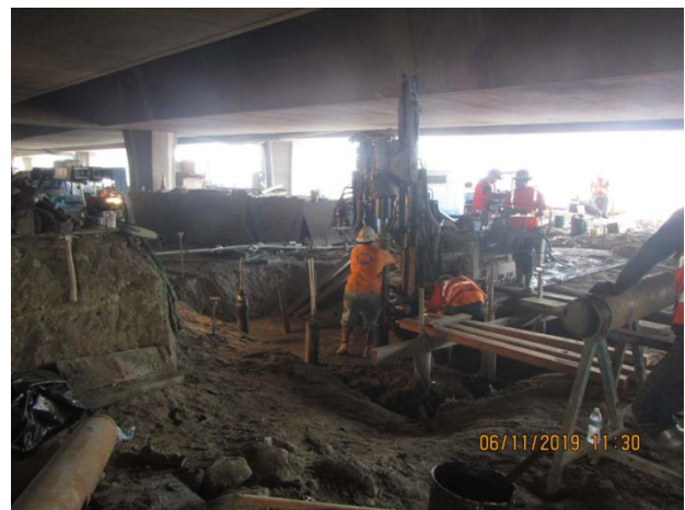
Bent 1 micropile drill operation
