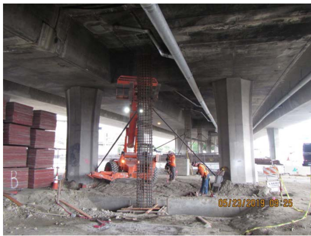
Setting rebar cage for C1
