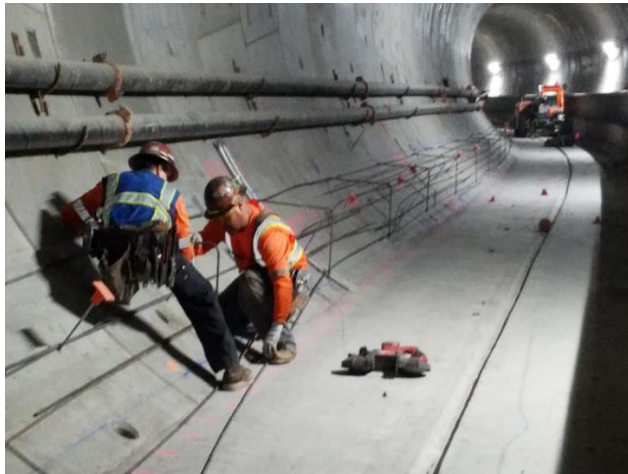
Formed Floating Slab Curb in left tunnel
