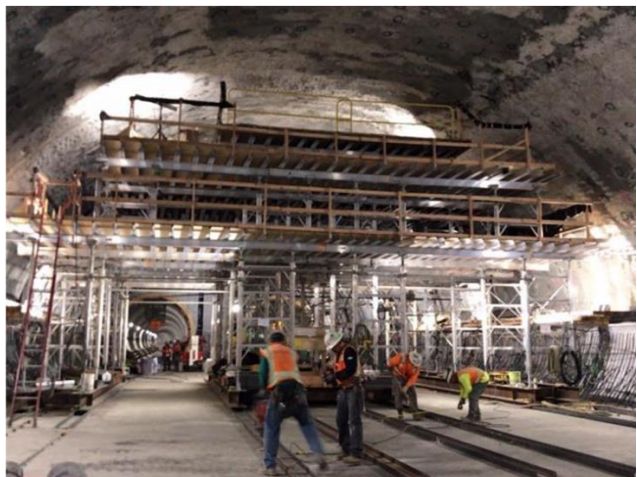
Scaffolding setup in SEM Cavern
