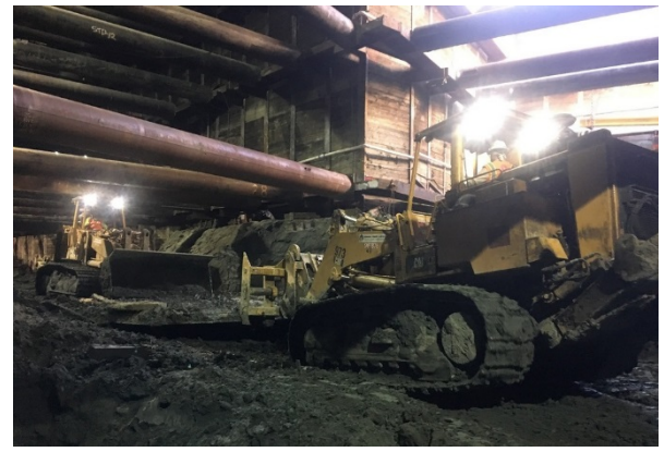
Wilshire/La Cienega Station Excavation
