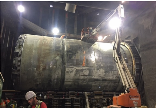
TBM Shield at Wilshire/Western
