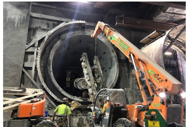
Reach 1 Tunnel at Wilshire/Western
