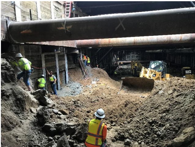
TBM Launch Box Excavation in Century City
