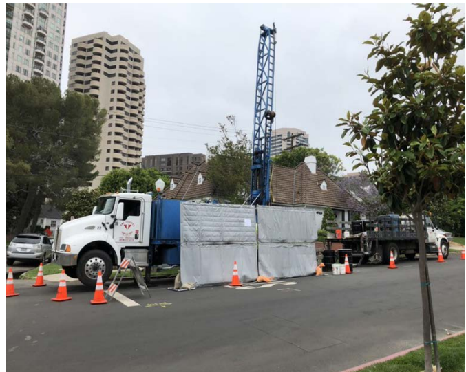
Geotechnical Boring R-19-015 Drill Rig Set Up of Sound Blankets
