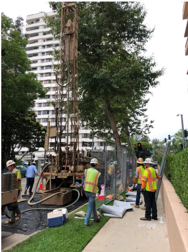
Geotechnical Boring R-19-017 Sound Blankets Installation and Rotary Mud Drill Setup
