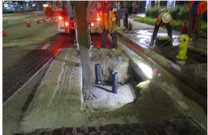
Backfill with Slurry Trench 10960 Wilshire Blvd.
