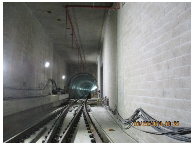
Transition to tunnel at Expo/Crenshaw Station
