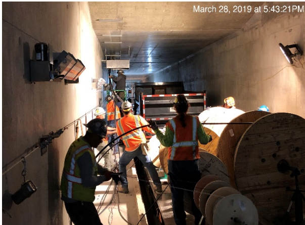
Install electrical conduit in underground tunnel
