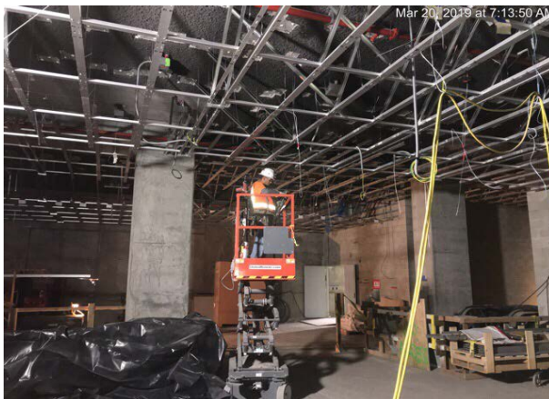
Installation of metal ceiling at Expo/Crenshaw Station
