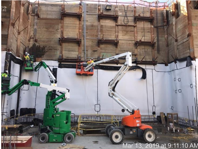
Water bar installation in future Little Tokyo/Arts District Station
