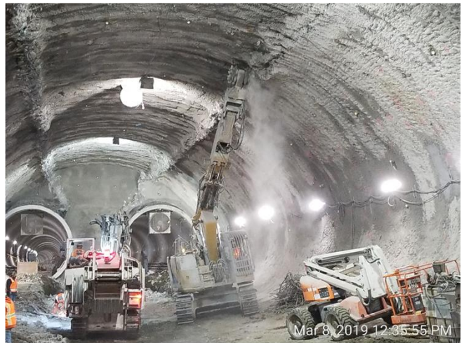
Wall grinding in SEM Cavern
