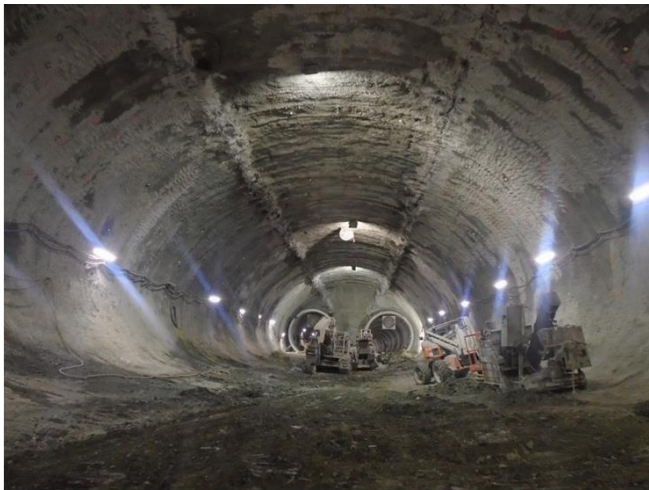
SEM Cavern excavation complete
