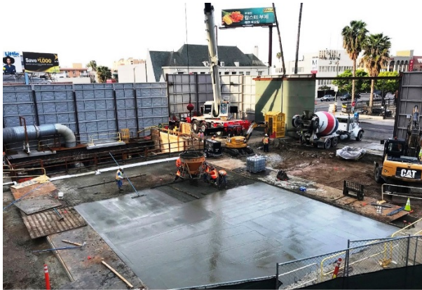
Gantry Crane Runway at Wilshire/Western
