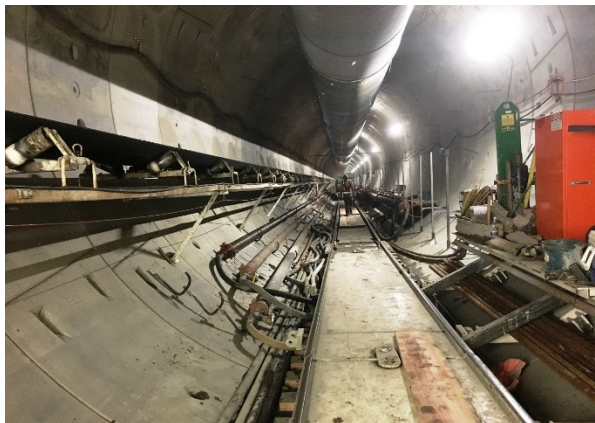
Reach 1 Tunnel Looking West
