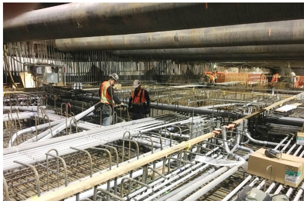
Wilshire/La Brea Station Conduit Installation
