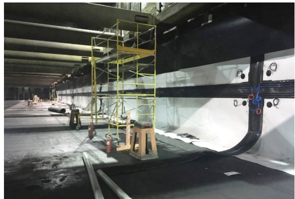
HDPE Placement at Wilshire/Fairfax Station
