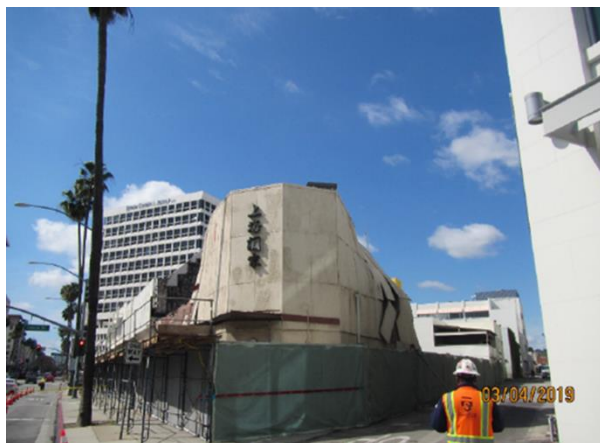
Demolition of North Canon Properties in Beverly Hills
