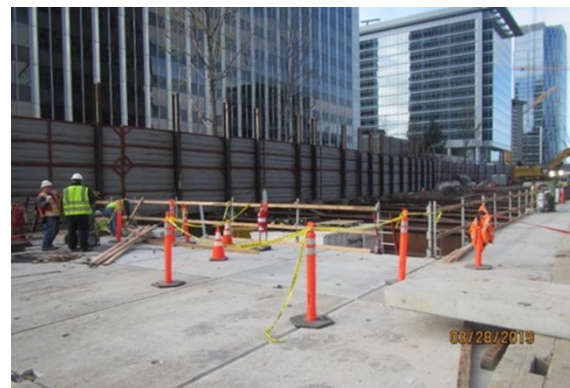
Installation of Temporary Deck Panels in Century City
