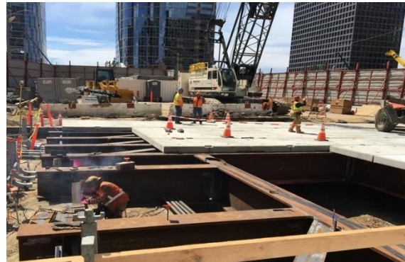
Installation of Deck Beams in Century City
