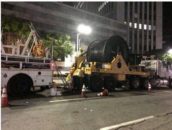
LADWP Cable Pulling
