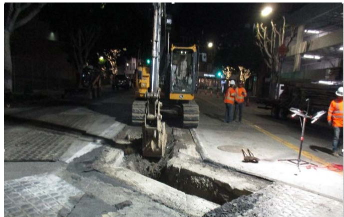
Water Line Excavation and Potholing
