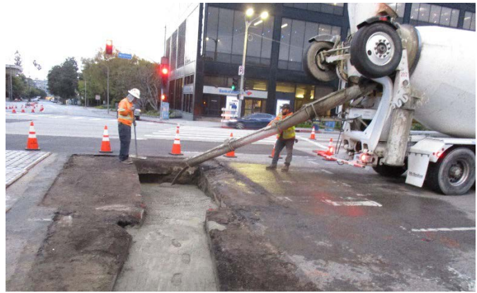
Utility Main Line A Slurry Backfill
