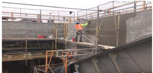
EXPOSITION/CRENSHAW STATION – Finishing coat at plaza walls.
