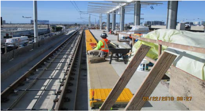
AVIATION/CENTURY STATION - tactile paver installation along platform.
