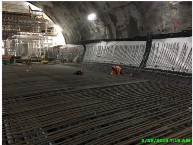
Rebar installation in SEM Cavern
