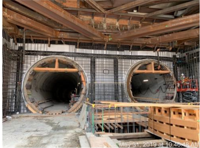
Rebar, MEP and formwork at future Little Tokyo/Arts District Station
