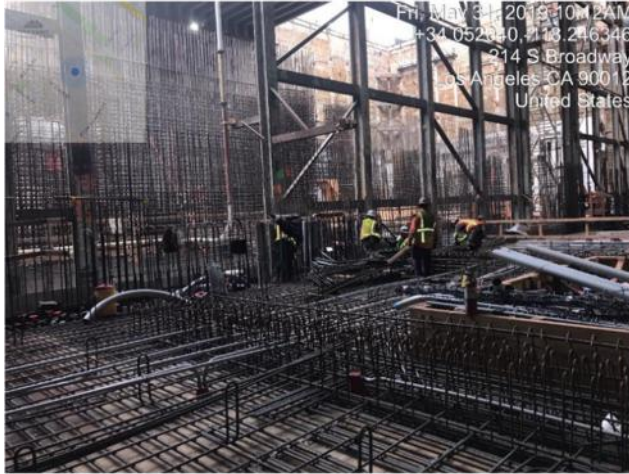
Systems work at Concourse Level of Historic Broadway Station
