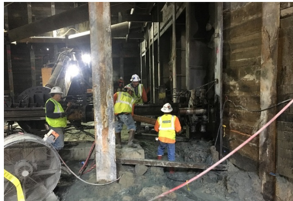
Pipe Canopy Work at Wilshire/La Cienega Station
