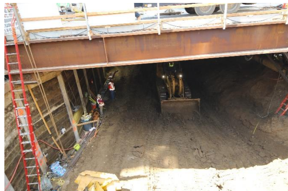
TBM Launch Box Excavation in Century City
