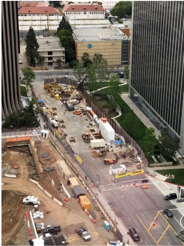
TBM Launch Box Overview in Century City
