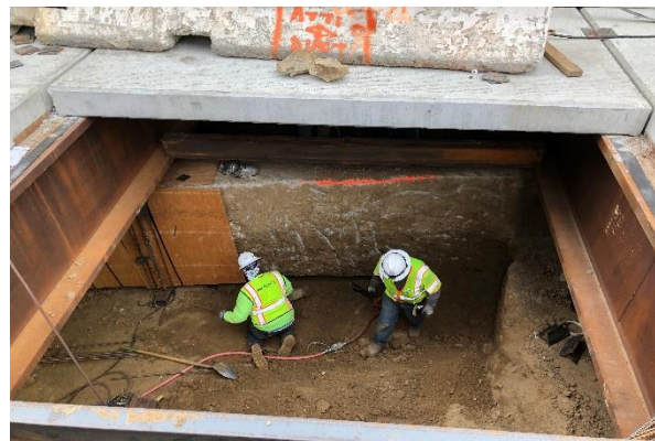
Utility Supported in Place in Century City
