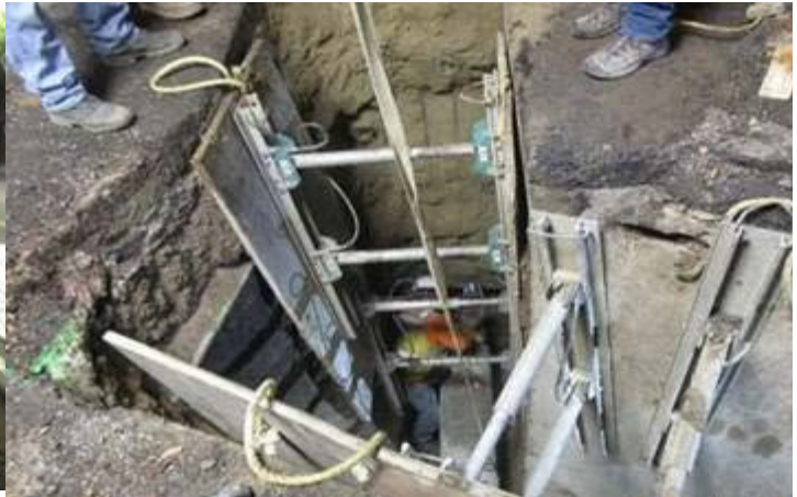
LADWP Water SWP Installation
