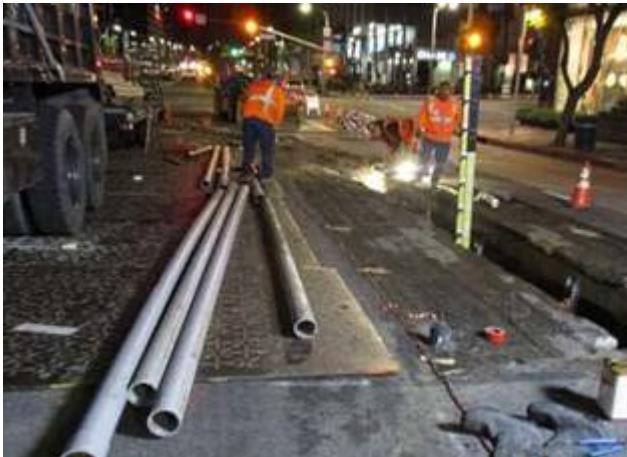
Joint Trench Conduit Installation
