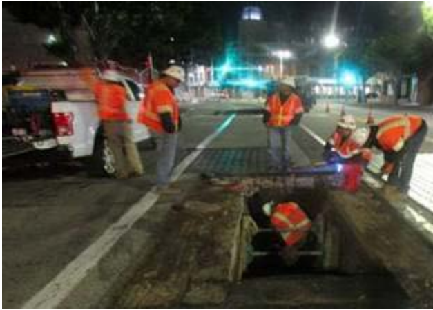
LADWP Water Riser Installation
