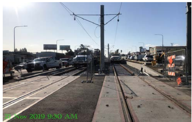
UNDERGROUND STRUCTURE #4 - Lineman preparing for wire run 31. 27 Nov 2019 9:30 AM
