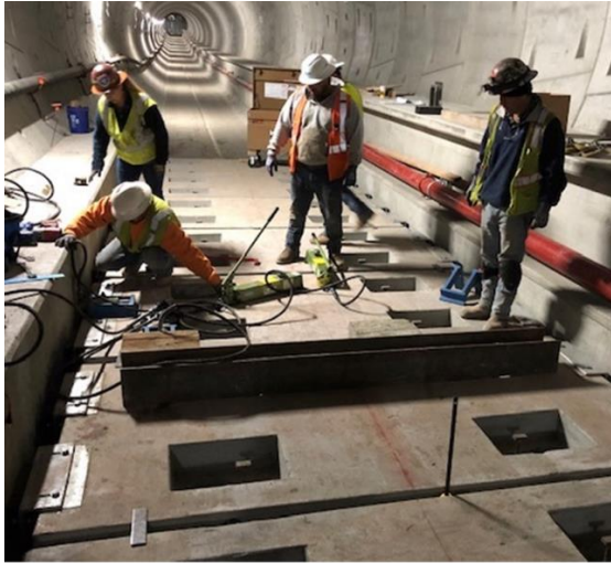
Floating Slab Track installation
