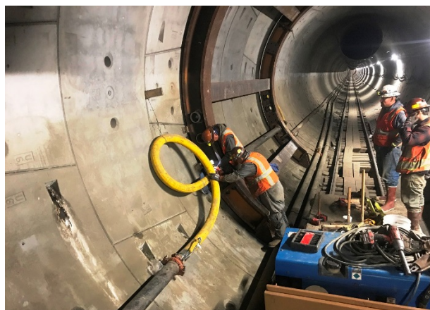
Work at Cross Passage 13
