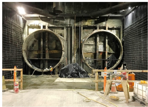
TBM Tunnel Eyes at Wilshire/Fairfax Station
