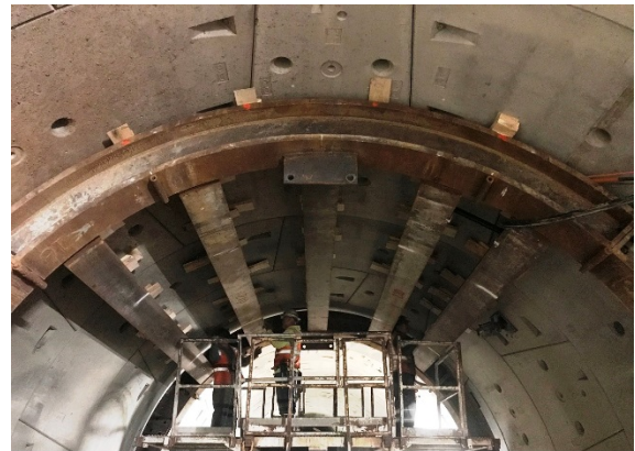
Support Ring Installation at Cross Passage 12
