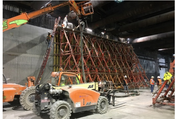
Exterior Wall Concrete at Wilshire/Fairfax Station
