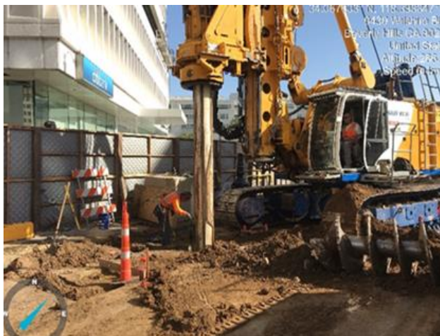
Wilshire/Rodeo Station Box Pile Installation in Beverly Hills
