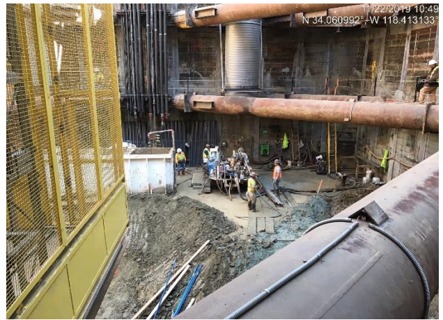
Tunnel Access Shaft Excavation in Century City
