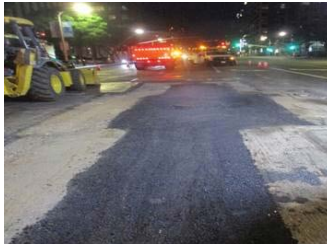
Telecom Joint Trench Lateral A13 Finished Base Paving
