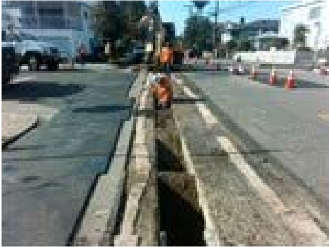
Excavation for the Gas line along Ohio Ave.
