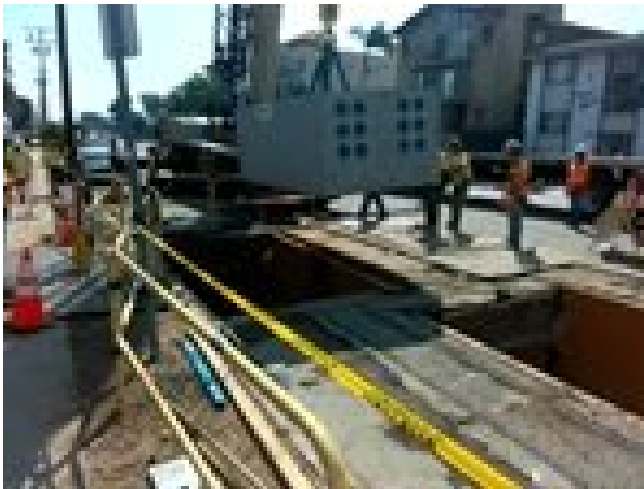
Install Manhole 500 for Conduit Line D
