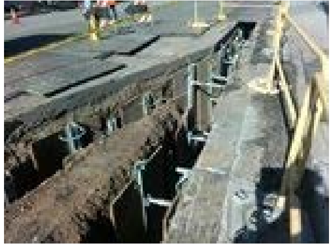
SCE Ductbank Trench Shoring
