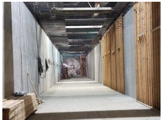
Left track tunnel at Flower St
