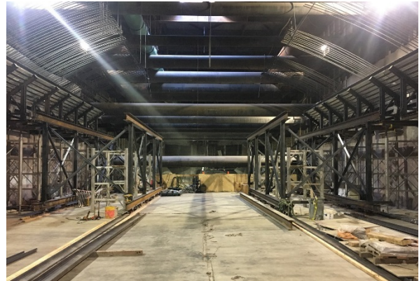
Roof Form Assembly at Wilshire/La Brea Station
