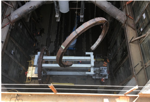
Lowering Tunnel Support Ring into Western Shaft
