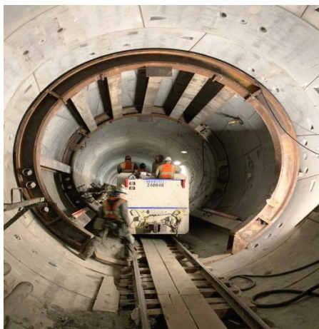
Reach 1 Cross Passage Excavation Preparation
