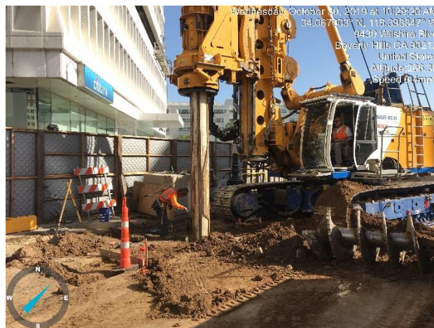
Wilshire/Rodeo Station Box Pile Installation in Beverly Hills
