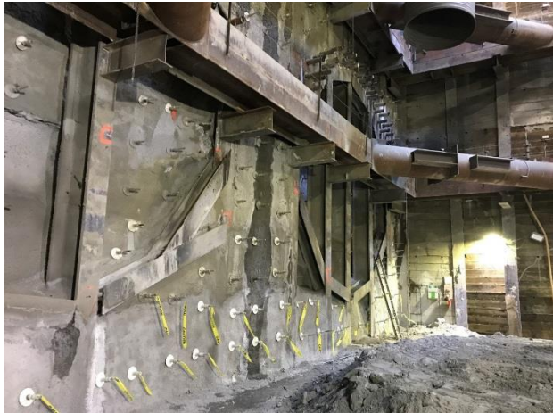
TBM Launch Box Excavation in Century City
