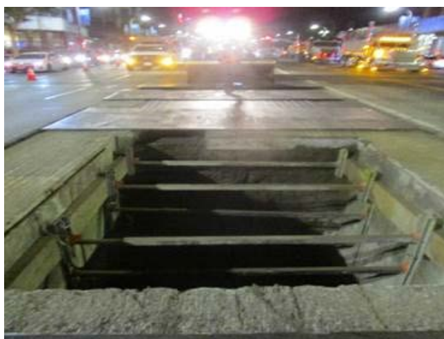
Telecom Joint Trench Excavation and Potholing Wilshire Blvd. and Westwood Blvd.
