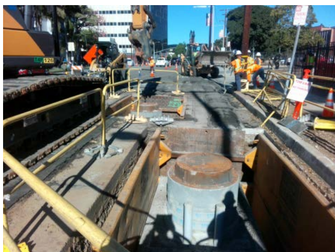
Install Manhole 500 for Conduit Line B
