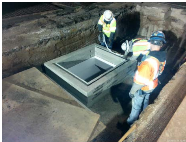
Install Grade Rings and Grout Neck Joints at Electrical Vault VLT-500
