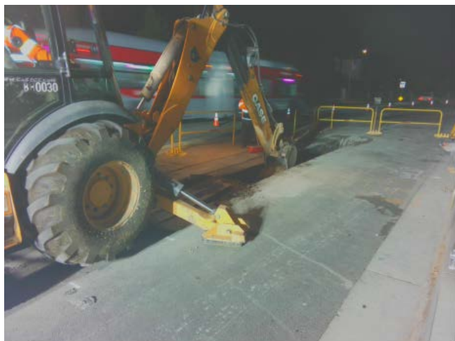
SCE Duct Bank Trench Excavation Along Wilshire Blvd.
