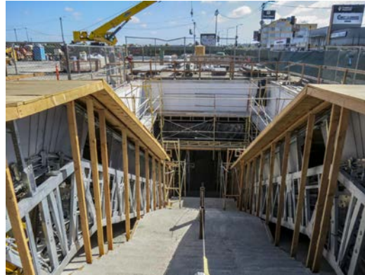
EXPO/CRENSHAW STATION – Plaza view at main entrance stairway.
