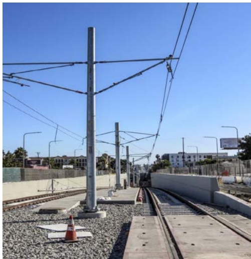
HYDE PARK STATION – Southbound view underground section transition.
