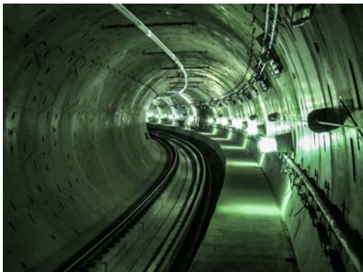
MARTIN LUTHER KING JR. STATION - Tunnel between stations.
