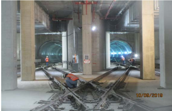
EXPO/CRENSHAW STATION – Track crossover section.
