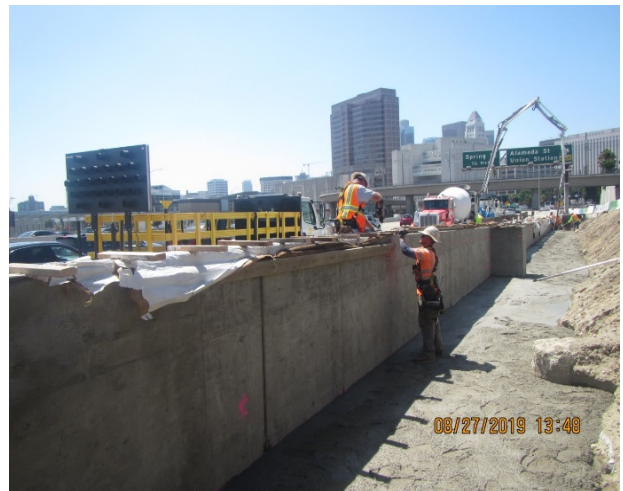
Backfill behind Retaining Wall 1
