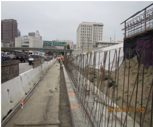
Pouring concrete at Retaining Wall 1 Footing
