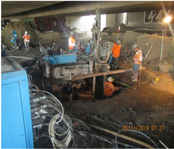
Two views of the Pedestrian Bridge Bent 1, 2, and 3 micro pile installation
