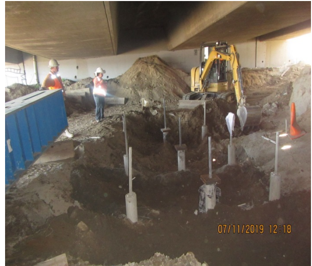
Two views of the Pedestrian Bridge Bent 1, 2, and 3 micro pile installation
