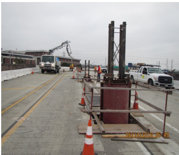
Pedestrian Bridge columns construction
