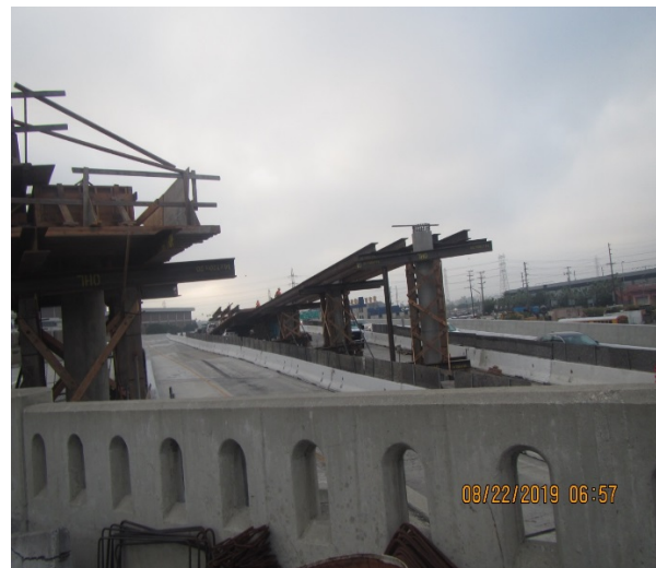
Falsework construction of Pedestrian Bridge bent cap 2
