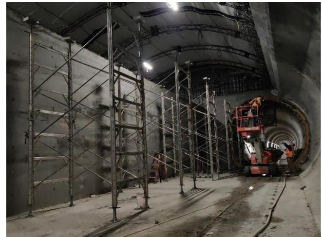
Installation of plenum deck shoring towers in SEM Cavern
