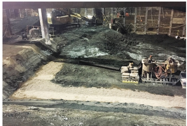
Wilshire/La Cienega Station Excavation
