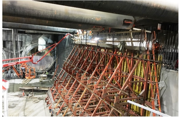
Concrete Placement at Wilshire/La Brea Station
