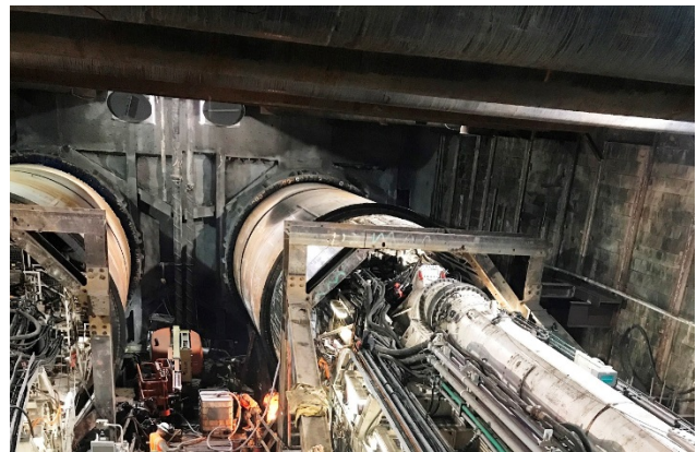
Preparing to Launch TBM at Wilshire/La Brea Station
