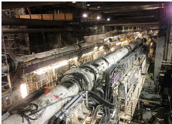
TBM Assembly at Wilshire/La Brea Station
