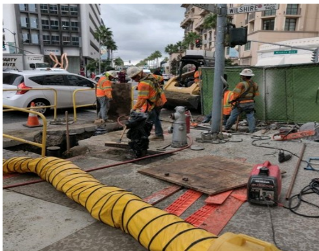
Utility Relocations in Beverly Hills
