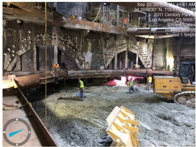
TBM Launch Box Excavation in Century City
