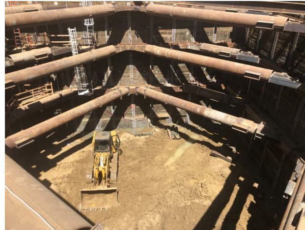
Tunnel Access Shaft Excavation in Century City
