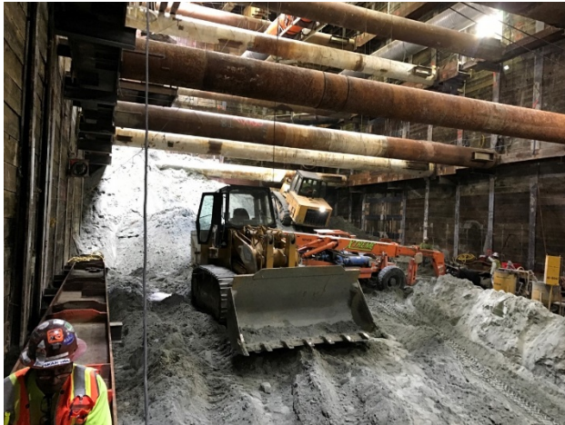
TBM Launch Box Excavation in Century City
