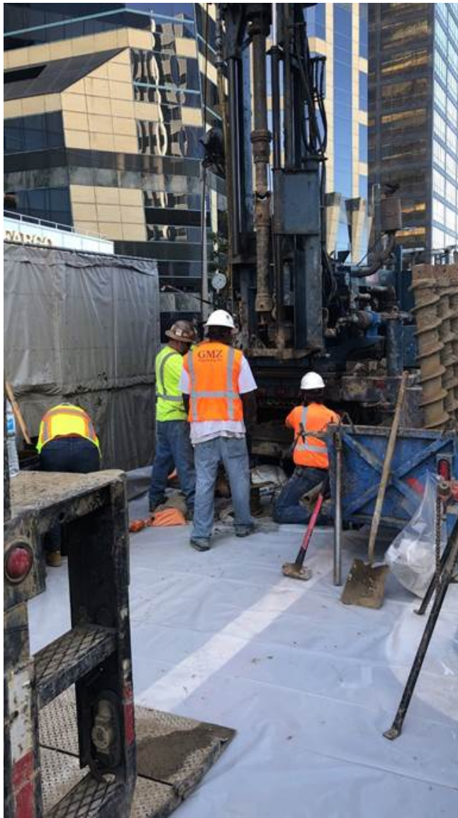
Installation of PVC Pipe for Well Development
