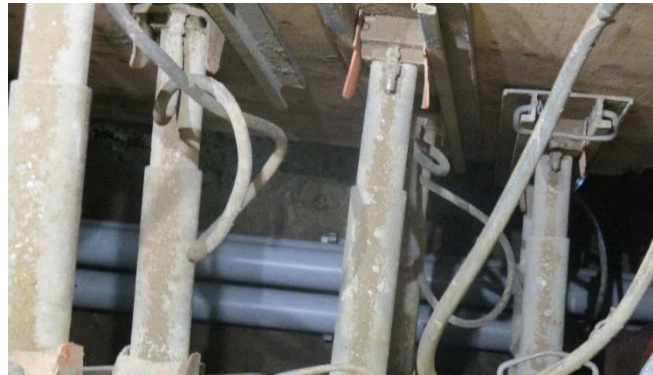
Lateral A5 and A7 Telecom Conduits Installed
