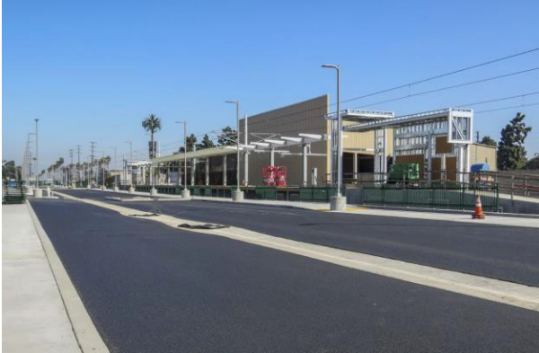
Fairview Heights Station – Station view, paved parking, sidewalks Lighting and fencing
