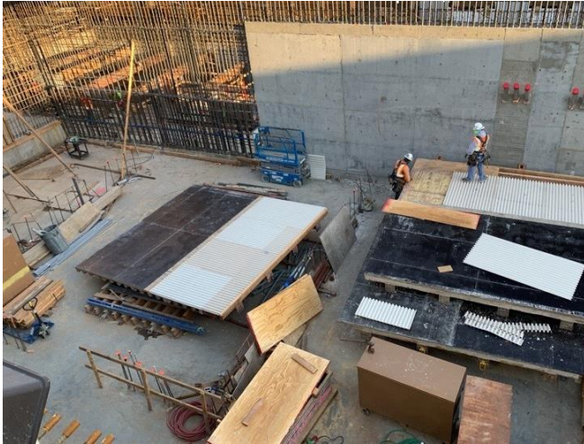
Wall form fabrication in future Little Tokyo/Arts District Station
