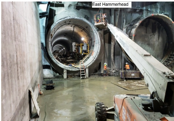
East Hammerhead at Wilshire/Fairfax Station
