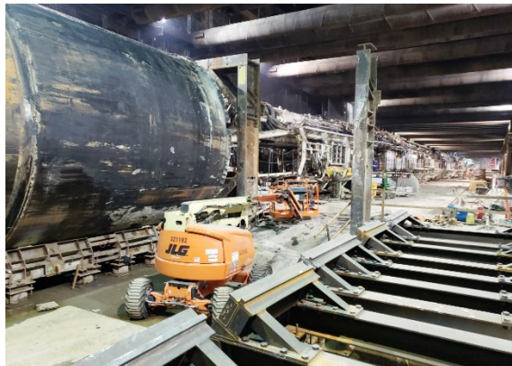
Purple TBM at Wilshire/Fairfax Station
