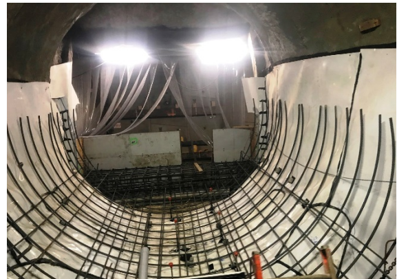
Installing Rebar at Reach 1 Cross Passage #10
