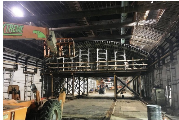
Roof Deck Shoring at Wilshire/La Brea Station
