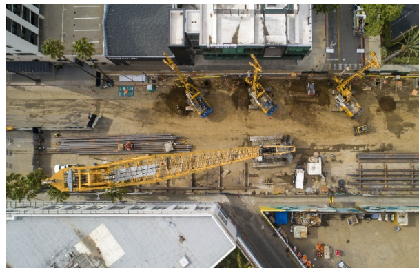
Wilshire/Rodeo Station Pile Installation During the Temporary Full Street Closure
