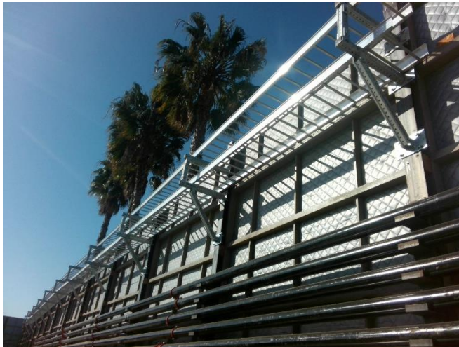
Cable Tray Installation on VA Soundwall at TTES Site
