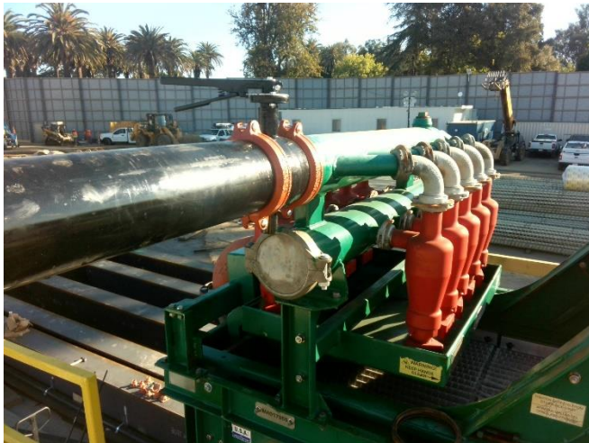
Separation Plant Inlet Line Installation at VA
