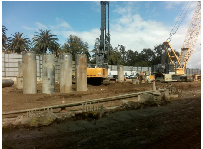
Drilling Operation at Pile S-9 at VA TTES Site
