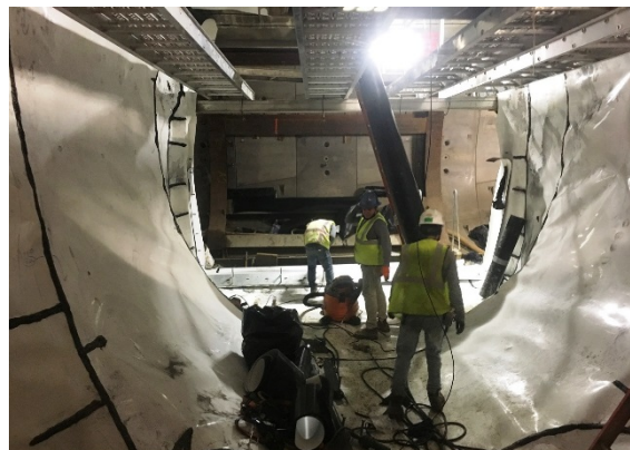
HDPE Installation at Cross Passage #8 (Reach 1)
