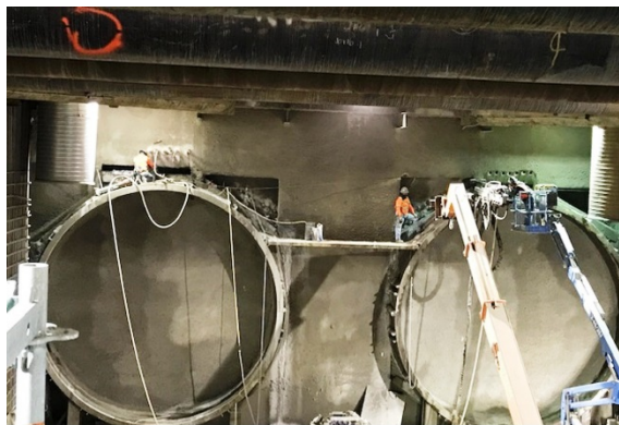
Grouting East End at Wilshire/La Cienega Station
