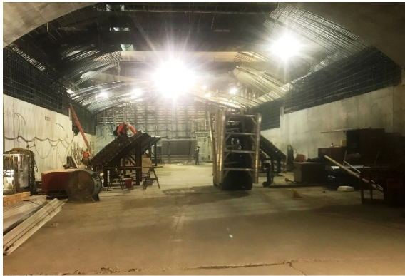
View of East Hammerhead at Wilshire/La Brea Station
