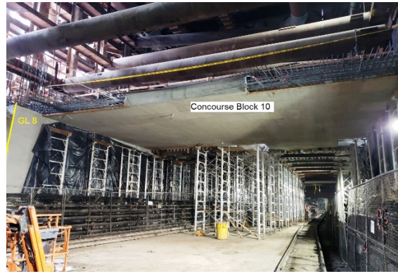
Stripping Concourse Shoring at Wilshire/Fairfax Station
